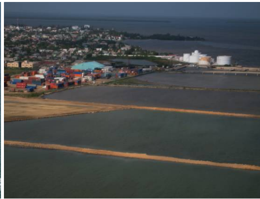
Construction site for the Carnival Cruise pier
